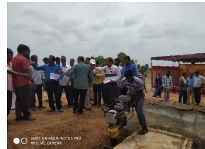
Compaction by Hand operated compactor at Sluice junctions
