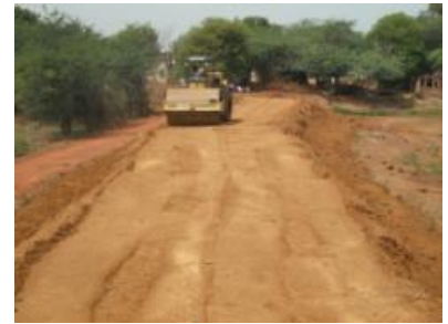
Compaction by Rollers
