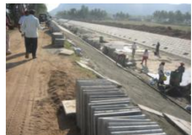
Side lining with precast slabs
