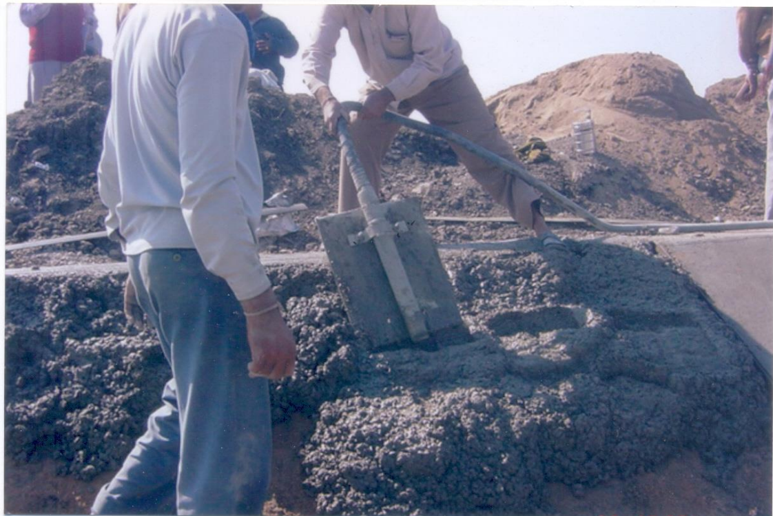
2. NEEDLE VIBRATOR CLAMPED ON STEEL PLATE
