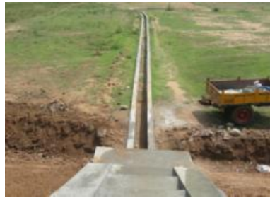
Lining of Channels below Sluice
