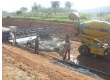
Bed Concrete with Pavers
