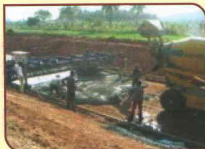
Bed Concrete with Pavers
