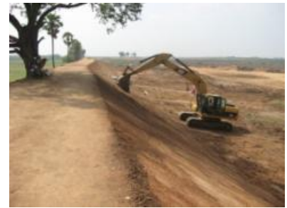
Side compaction by Plated Poclains
