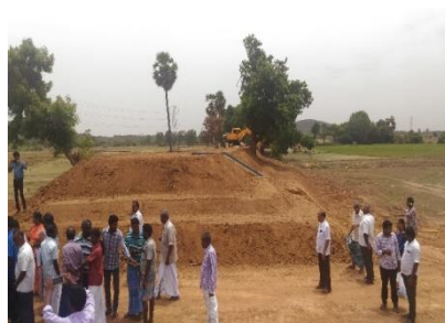
Benching along Cross Section
