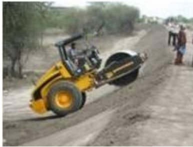
Side compaction by Vibratory power roller
