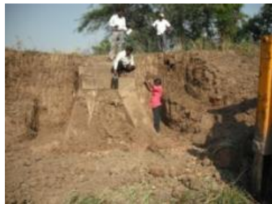
Dismantling dilapidated Sluice
