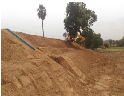
Benching along Longitudinal Section
