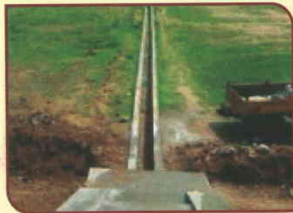
Lining of Channels below Sluice
