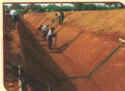
Lining of Canals – Gravel backing
