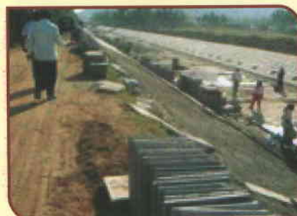
Side lining with precastslabs
