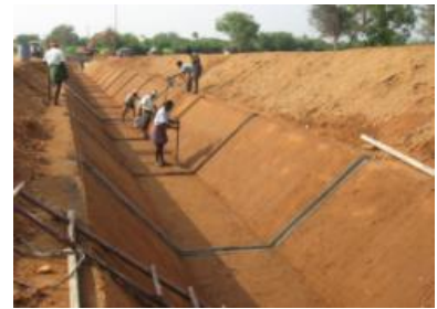
Lining of Canals – Gravel backing
